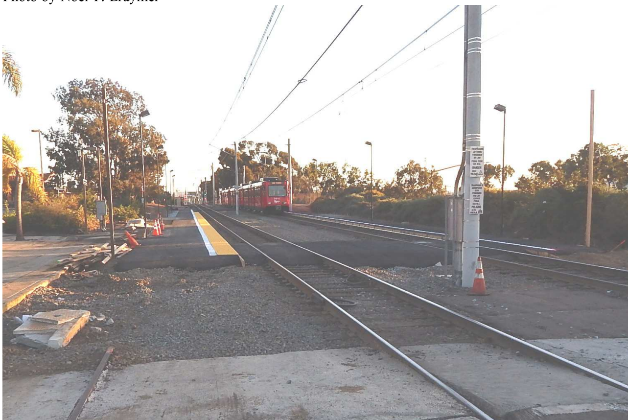
These are temporary platforms at the E Station Station which will be used while new permanent platforms are built where the old platforms are. With raised platforms, new low-floor Trolleys can be used for easier and faster access for all passengers. Photo by Noel T. Braymer
