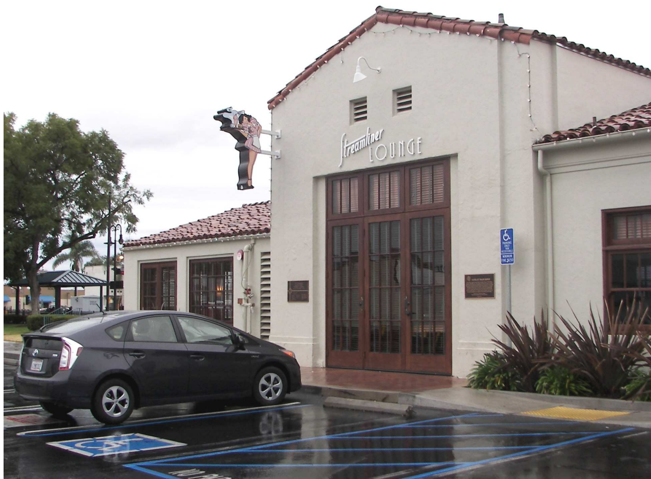
This is the old ATSF Station building at the City of Orange Metrolink Station. The station has a Ruby's Diner with it's own Streamliner Lounge. Photo by Noel T. Braymer
