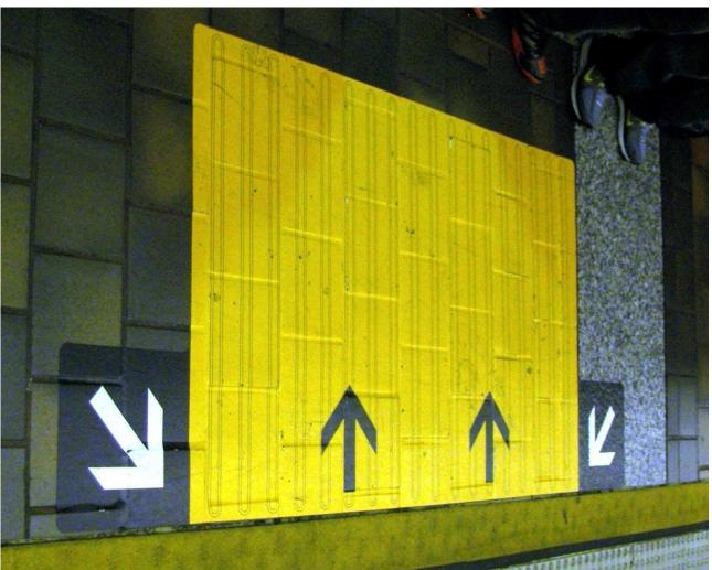
What in the world is this??? You might ask. This is one of the/ experimental mats that have been placed at the 7th and Flower St subway station in Los Angeles to speed up loading. The yellow area on the platform is next to the doors of the subway cars and the black arrows shows the way out for exiting passengers. The white arrows show where boarding passenger should wait while the train passengers unloads before boarding. Photo by Noel T. Braymer
