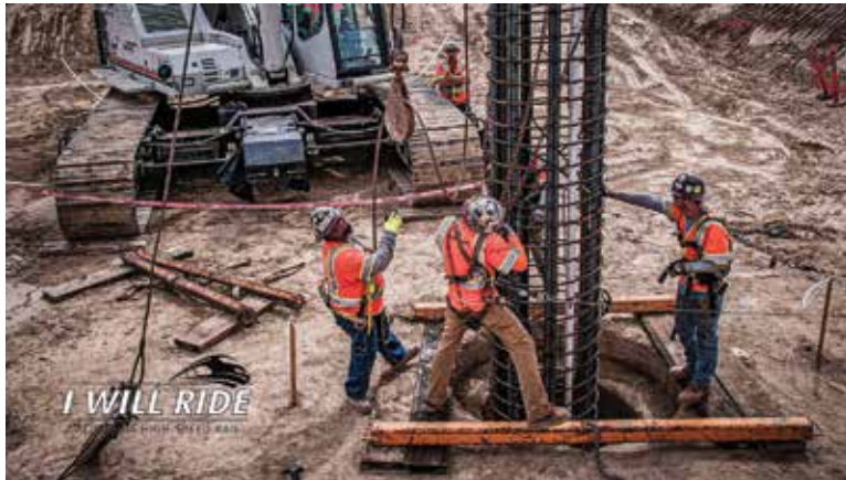
HSR Crews at work 2021 Photo courtesy of CHSRA
