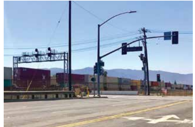
Existing McKinley street grade crossing of BNSF mainline in Corona
