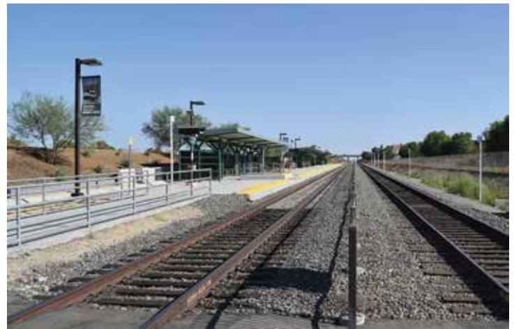
Moreno Valley/March Field station, on the Perris Valley Line
