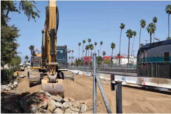
Riverside-Downtown Station Layover Facility, under construction in mid-September 2020
