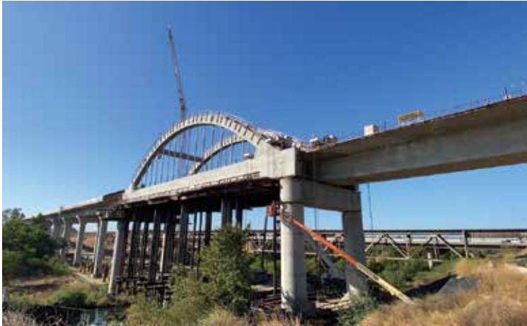
San Joaquin River Viaduct - July 2020 Pictures courtesy of CHSRA
