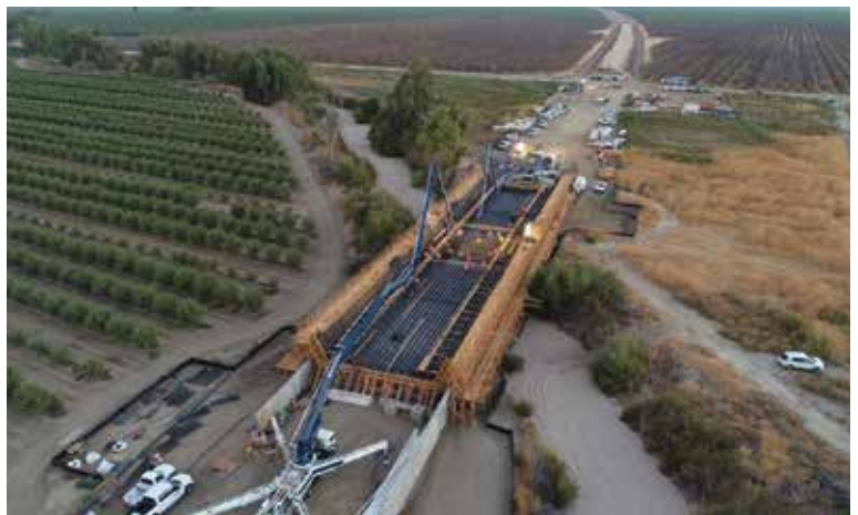
Poso Creek Viaduct - July 2020 Pictures courtesy of CHSRA
