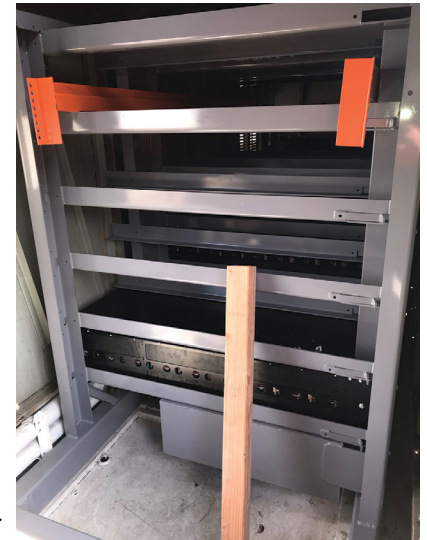
RPS designed and built racks for the Lithium Iron Batteries for the second battery prototype. The batteries are recycled from “Mini-E” electric cars. Photo Credit: Brian Yanity
